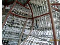
Visually interesting, the mass of each curved surface isolates each space acoustically. Curved-Right® framing elements help support 3" shot crete, 1 layer of varnished MDF, and 2 layers of gypsum wall board.
