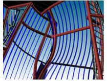
Radius Track Corporation designed each unique framing assembly for the office and rehearsal spaces where Ninety-four percent of the curved framing members fabricated are one-of-a-kind including the knife edges.
