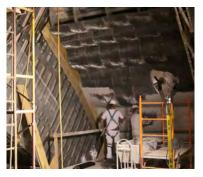
Behind the acoustically transparent metal mesh, convex reflective surfaces in 3 sizes, small medium and large, prevent acoustic focus and provide diffusion of sound to all seats in the audience.
