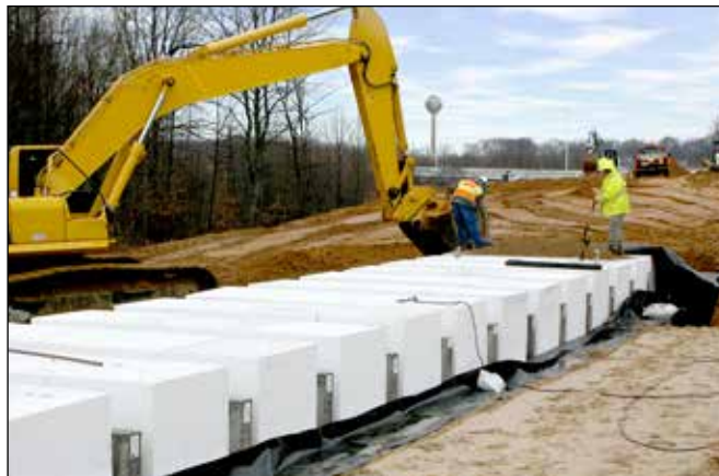
EPS Geofoam Protection
