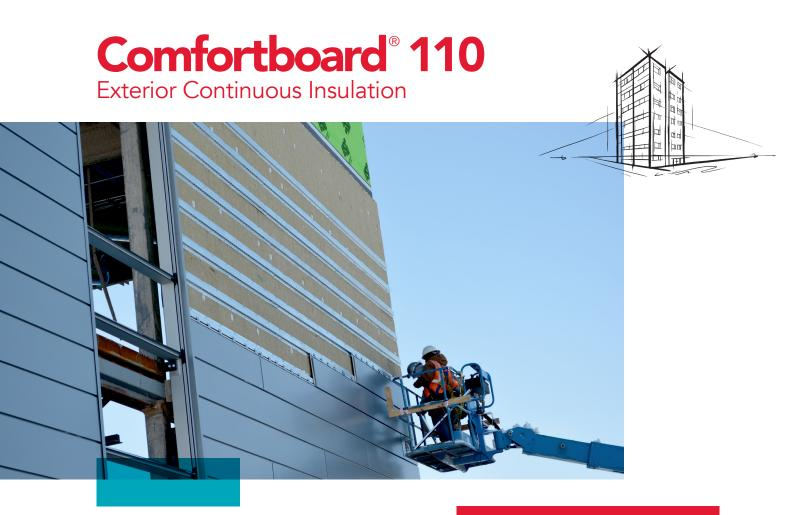
ROCKWOOL Comfortboard® 110 is a rigid, high-density, noncombustible stone wool insulation board designed for use as an exterior continuous insulation in commercial applications.
