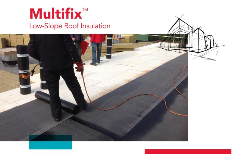
Multifix™ is a rigid, high-density stone wool insulation product with a mineral-coated fiberglass facer that is compatible with multiple attachment methods including torched, hot-mopped, cold-adhered and liquid systems.
