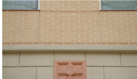
The block, accent medallion and running bond appearance (with darker stretcher bond accent rows), are all done in EIFS.
