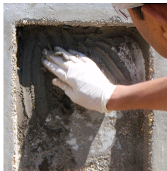
Moist cure and protect from elements immediately after finishing.
