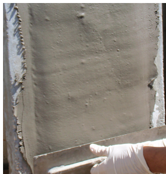
Scrub material into substrate, filling any pores and voids.
