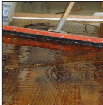
Spread material using a 3/16" notched squeegee.
