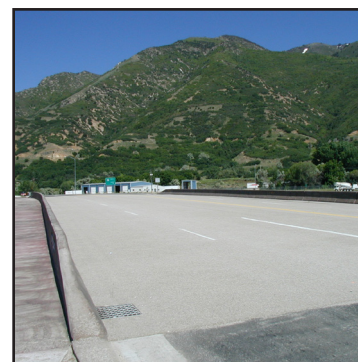
Remove excess aggregate after epoxy has set.
