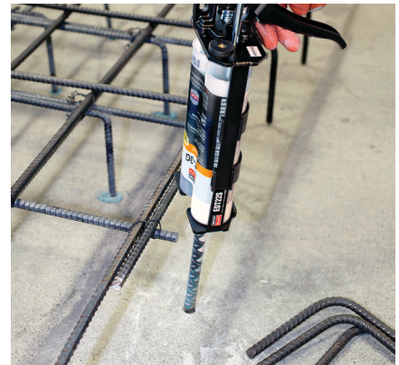
ET-3G Rebar Installation
