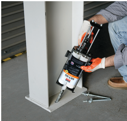
SET-3G — Column Installation
