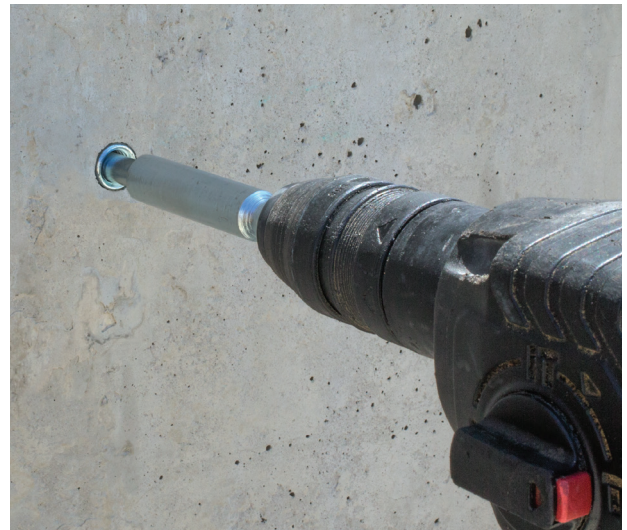
Anchor being set with SDS setting tool.
