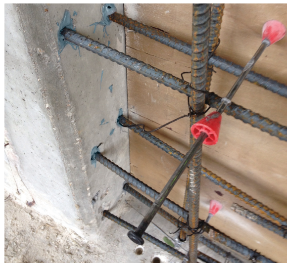
Rebar Wall Extension
