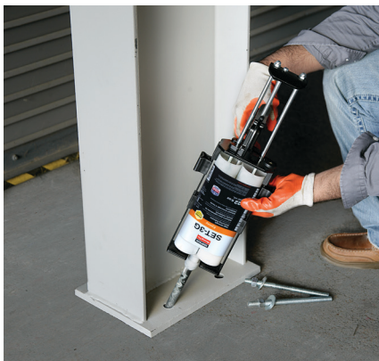
SET-3G — Column Installation
