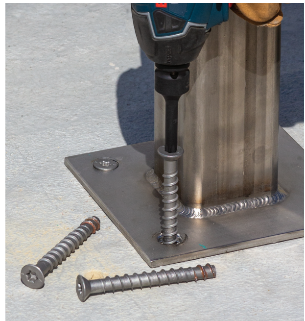
Titen HD Countersunk Installation
