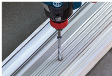
Sliding door track installation
