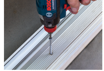
Sliding door track installation
