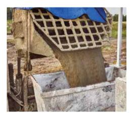
**STEP 3** Once all the materials are in the mixer allow 4-5 minutes mix time. Before dispensing the mortar into your tub, if the mortar is not the desired consistency or flow, only add additional water for optimal workability. Use mortar within 2.5 hours after initial mixing.
