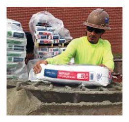
**STEP 2** Next empty one 80 lb (36.2 kg) bag of SPEC MIX® Masonry Mortar into the mortar mixer. NOTE: Mixing mortar by hand can cause mortar color inconsistency. Only add additional water to stiffened mortar lost due to evaporation.
