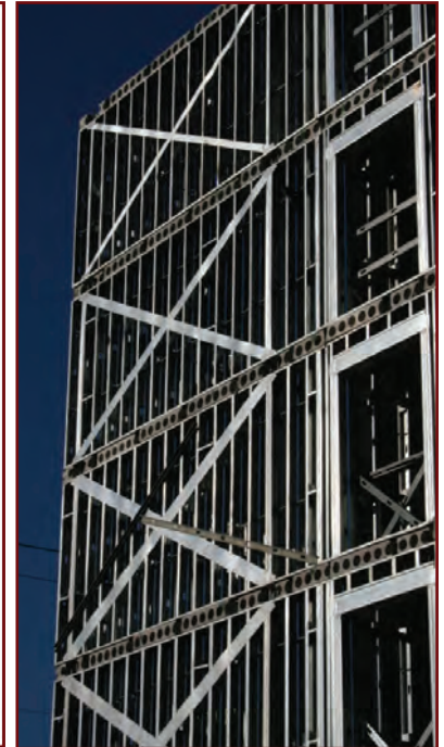
Fig. 3: Shear walls should be stacked vertically.
