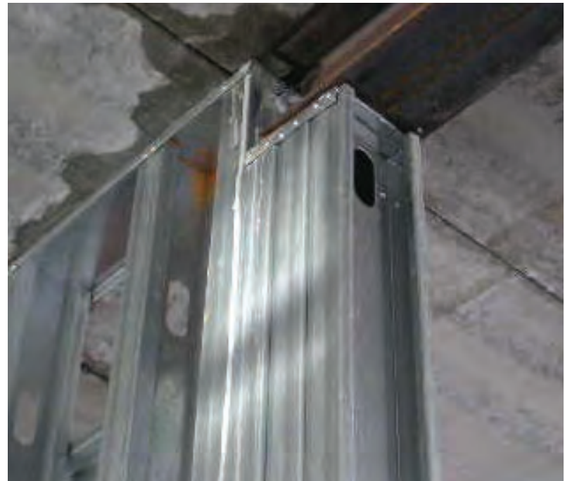
Picture of corridor framing, with SigmaStuds supporting the distribution lintel.
