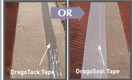
At a Location Designated by the Design Team: Seal Drago Wrap to concrete with DragoTack Tape or DragoSeal Tape .
