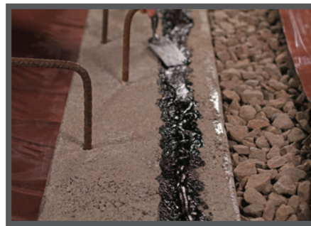
Onto Interior Grade Beams at Impediments: Seal Drago Wrap to concrete with Drago Mastic .
