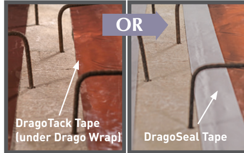
Onto Interior Grade Beams at Impediments: Seal Drago Wrap to concrete with DragoTack Tape or DragoSeal Tape .
