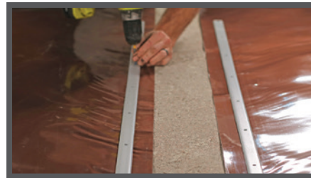
Onto Interior Grade Beams at Impediments: Seal Drago Wrap to concrete with DragoTack Tape or DragoSeal Tape .
