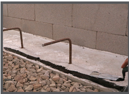
Onto a Perimeter Footing at Impediments: Seal Drago Wrap to concrete with Drago Mastic .
