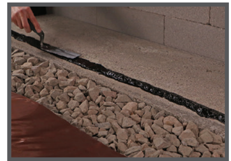
At a Location Designated by the Design Team: Seal Drago Wrap to concrete with Drago Mastic .
