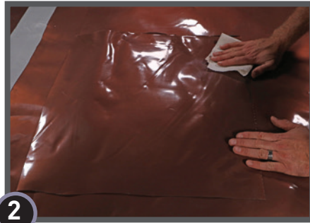
2 Measure and cut a piece of Drago Wrap to cover damaged area 6" in all directions. Clean area of adhesion.
