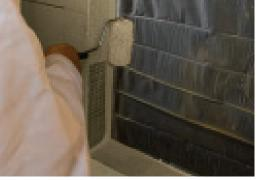
2. Embed fabric into Sto EmeraldCoat®. Be sure it overlaps the StoGuard RediCorner by two inches (50 mm) minimum.
