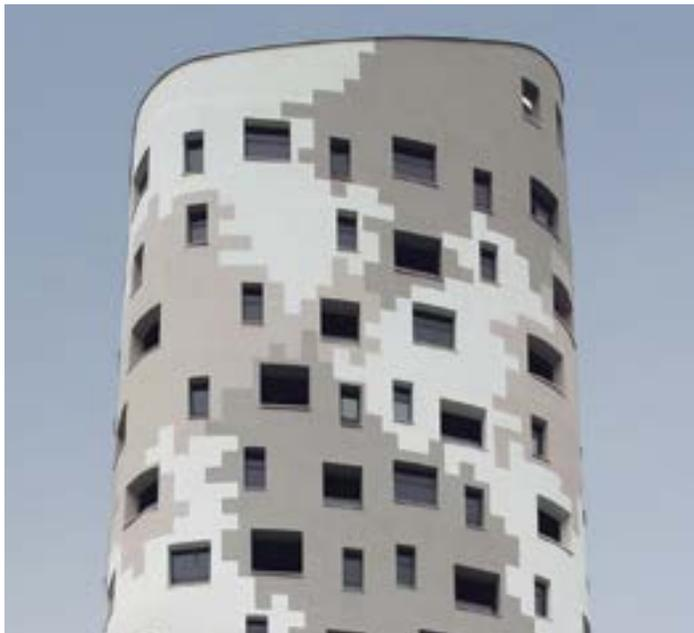
This design flexibility is taken to its fullest potential when the possibilities of StoVentec Sub-construction are utilized. The adjustable StoVentec Sub-construction not only makes substrate imperfections easy to manage, it can also be formed and adjusted to create unique curved surfaces, making use of the flexible nature of StoVentec Carrier Board A+.
