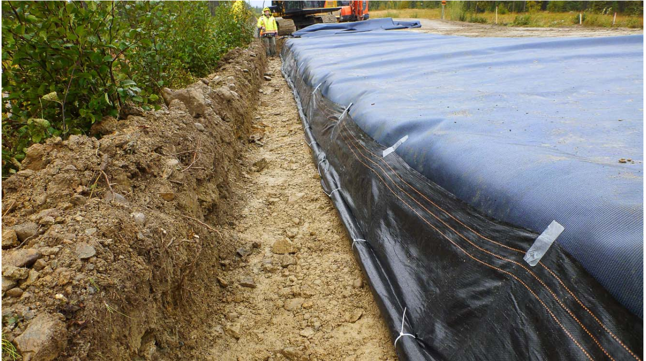
Image 12 - Pipe Installation with Separation Geotextile
