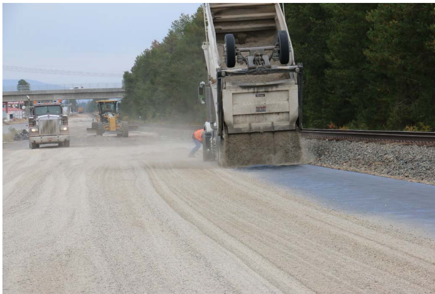
Photo 17. Gate Set to Spread 1" (25 mm) Lift Allowing a Full Spread Over One Roll.
