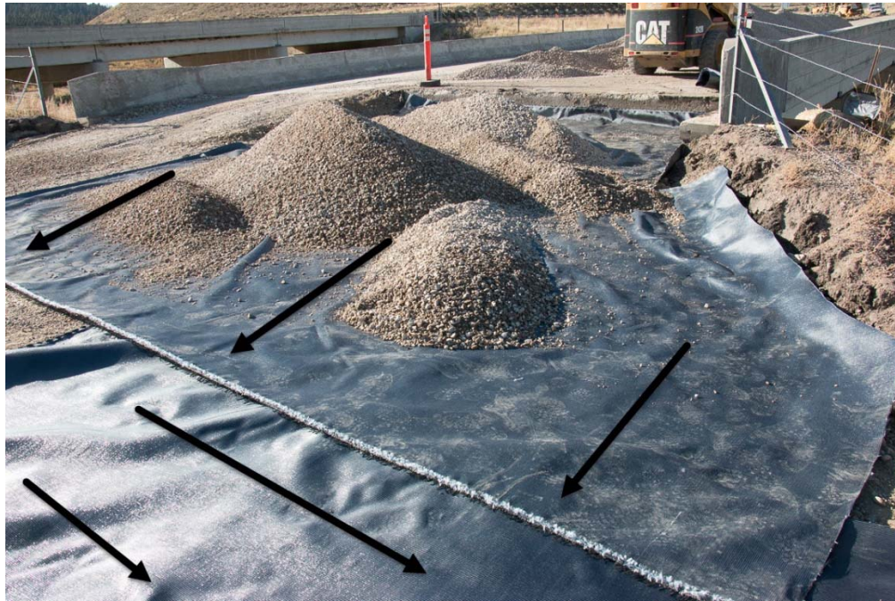
Image 5 - Bridge Approach, Routing Water Away from Structure.
