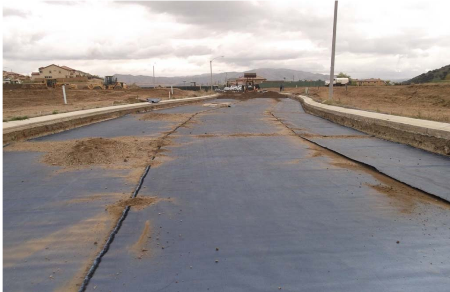
Image 7 - Traditional Installation with No Outlet
