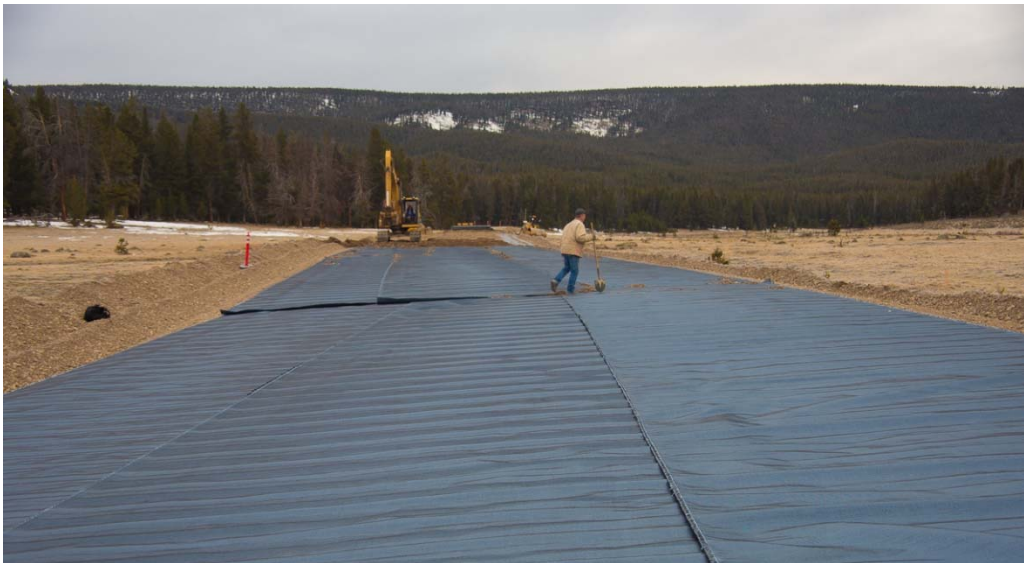
Image 4 - Installation Through Super-Elevation on Right, Moving Water from Right to Left
