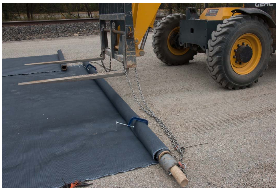
Image 15 - Clamps Used to Secure the Material to the Core
