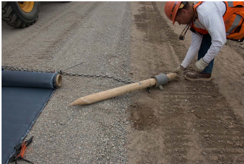
Image - 14. Fence Posts Used as End Holders for Unrolling
