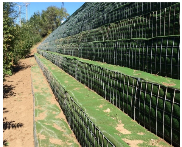
Figure 6(b): Project photo of WWM with MIRAGRID Miramesh GR during construction
