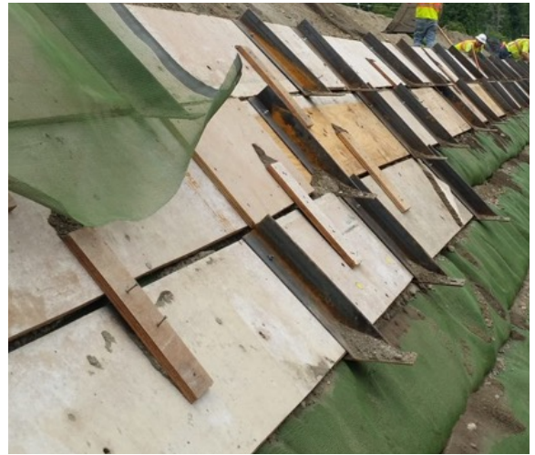
Figure 7(b): Project photo of MIRAGRID Miramesh GR face wrap installed with a temporary wooden form with a face batter angle [as opposed to the stepback typical detail shown in Figure 7(a)]
