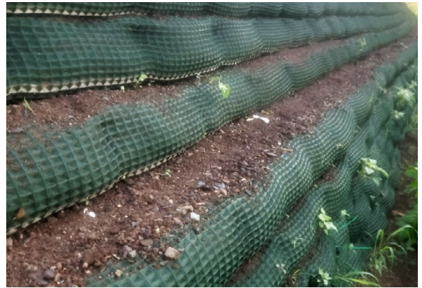
Figure 9(b): A completed PROPEX Pyrawall installation
