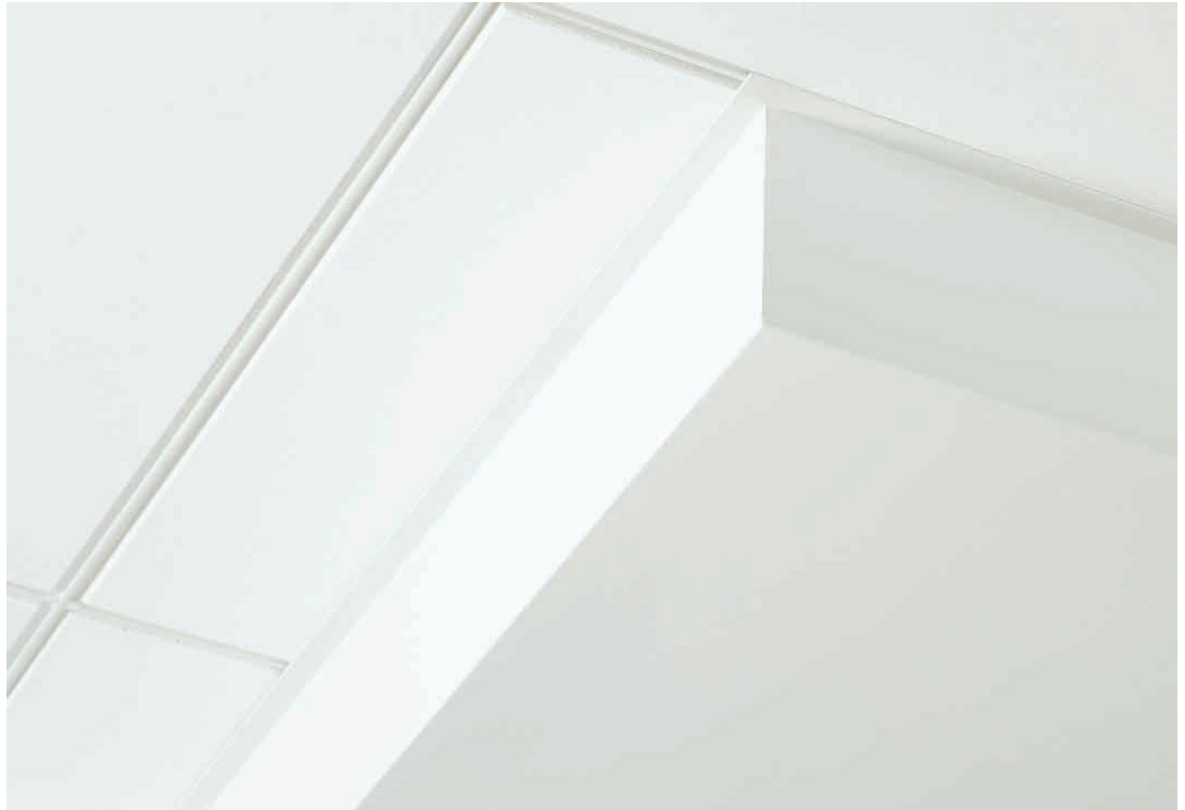
Elevation - USG Compässon™ Elite Drywall to Acoustical
