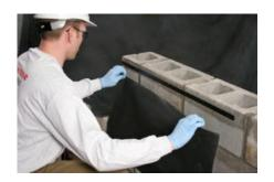
**Step 3**- Attach the EPDM membrane to the wall. Continue the membrane down the wall, continue over the wall-to-footing transition and continue out to within 0.5" (1.27 cm) from the edge of the brick shelf.
