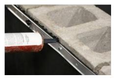
**Step 6**- Place a continuous bead of Sealant along the top of the termination bar and over the exposed fasteners.
