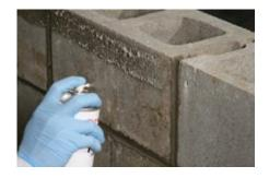
**Step 1**- Spray the substrate and membrane with an Spray Adhesive/Primer and allow it to dry. Drying time is typically 2 – 3 minutes depending on ambient temperatures.
