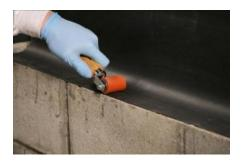
**Step 8**- Secure the membrane to the brick shelf. Roll with a 1.5" (3.81 cm) roller to insure complete contact.
