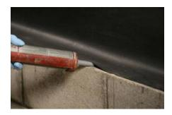
**Step 7**- Place a continuous bead of Sealant within 0.5" (1.27 cm) of the outside edge of the brick shelf.
