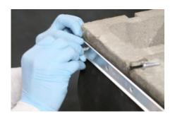
**Step 4**- Place the termination bar or strip aligned with the top of the membrane.
