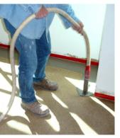
A standard traffic-grade, single-component, volumetrically-stable, self-leveling floor topping and underlayment that may be pumped or poured.
