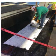
HRM 714 is hot-applied to form a continuous elastomeric membrane. It is ideal for waterproofing bridge, parking, plaza, or promenade decks; tunnels; pedestrian concourses; and similar types of construction where a monolithic waterproofing membrane is desirable.
