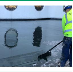
HYDRALASTIC 836 SL self-leveling waterproofing system is created from a single-component, moisture-cured, liquidapplied compound that will not shrink or crack.
