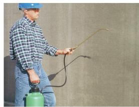
VOCOMP-20 waterbased curing and sealing compound may be quickly and easily applied to simultaneously cure and/or seal new interior or exterior as well as vertical or horizontal surfaces.
