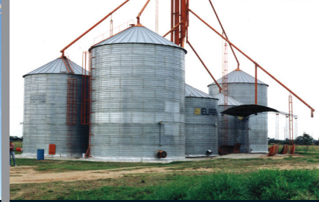
Calafate S.A. Cereal Storage Silos, Argentina
