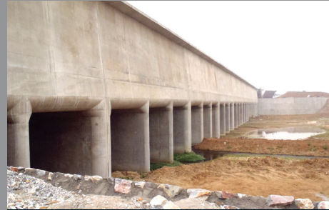
South-North Water Transfer Project, China
